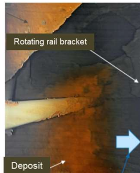
Photos taken from investigation inside the Unit 3 pedestal (Reference: the TEPCO Holdings website)
