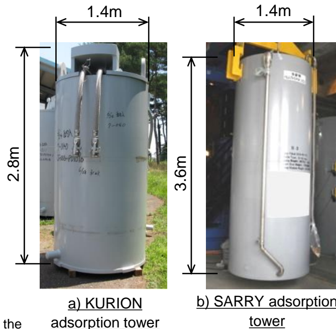
Figure 2 External appearance of adsorption tower
