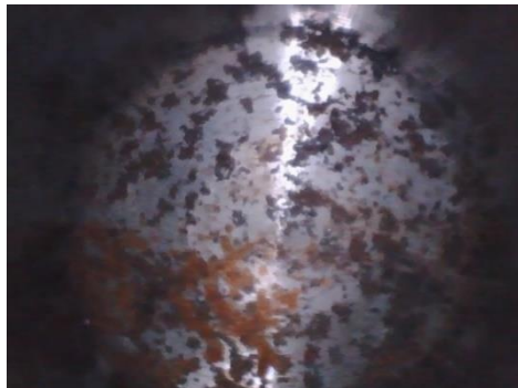
Condition of the surface of the flange before making an opening
