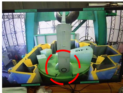
Figure 2 Camera image while verifying whether the hook of the adsorption tower is set
