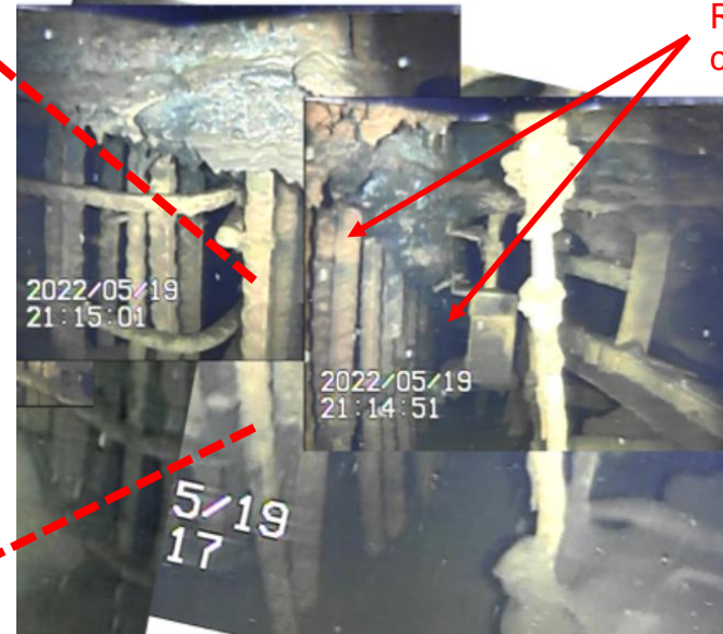
Photo 2: Concrete remains seen from the pedestal opening
