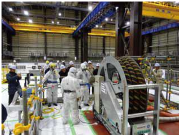
Verification test of strengthening workability of the S/C support column
