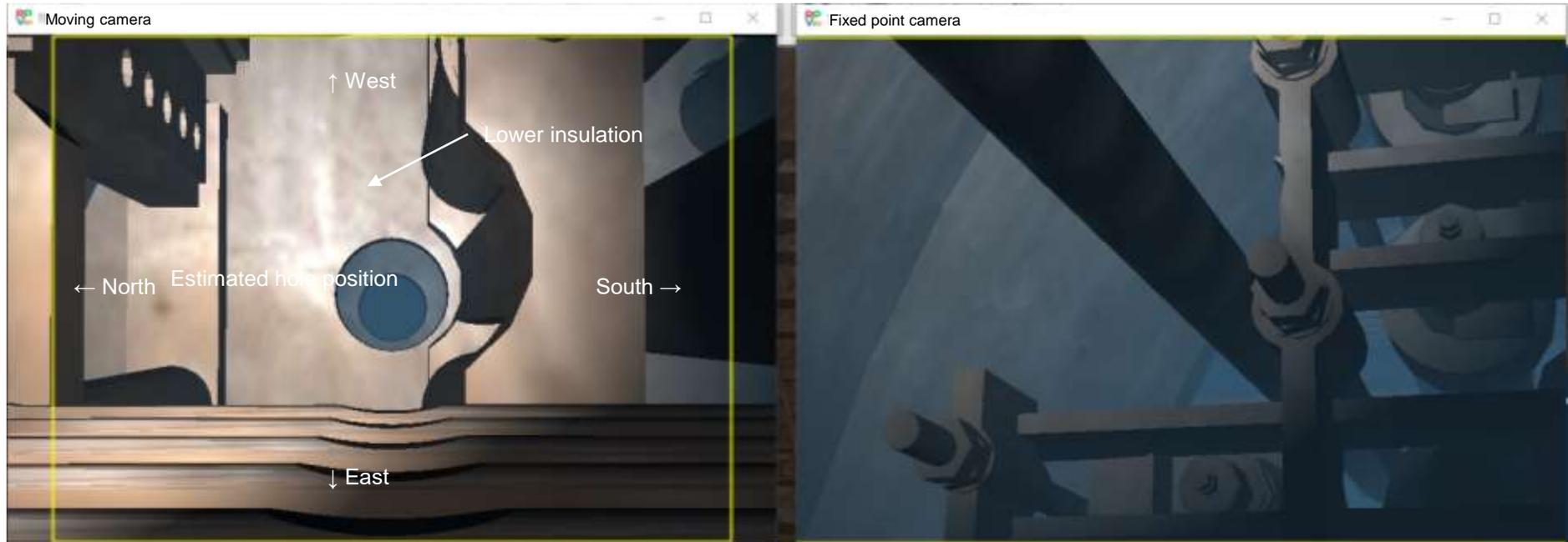
Unit 2: Camera image with telescopic pipe extended 2000 mm from retracted state (tilted 2° to the west)
