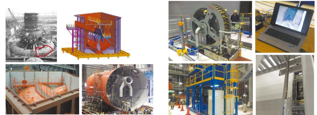
▲ Upper left: primary containment vessel (when building Unit 1; simulated S/C is in the red box); Upper right: full-scale S/C (1/8 sector) CAD drawing; Lower left: vent pipe and S/C; Lower right: assembled S/C shell and downcomer (Photo 1)
