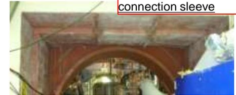
After removing the concrete block (Fukushima Daiichi NPS-4 X-1B)
