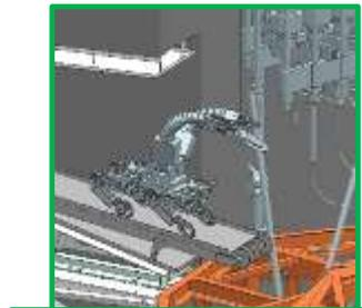
Illustration showing removal of interfering objects from around the CRD opening
