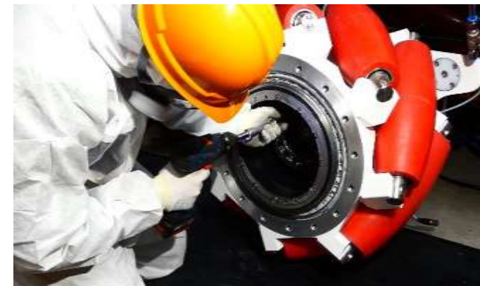
Photo 7 Maintenance test (replacement of travel motor)
