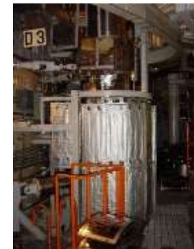
Figure 14: View seen from B (PLR shielding: before the earthquake disaster)
