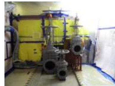
Figure 13: View seen from A (access route)
