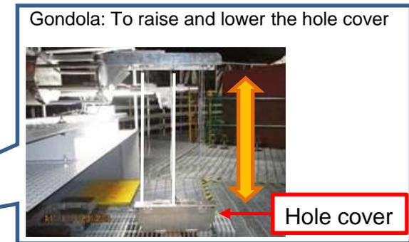
Hole cover: Transported in a folded state, and spread out at the time of installation to close the hole for ROV.
