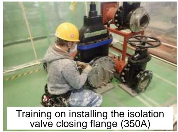
Training on installing the isolation valve closing flange (350A)
