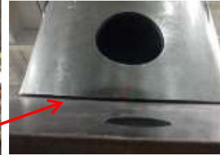
Condition of extension pipe - S/C surface after positioning (No.8)
