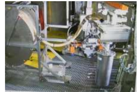
Recovery of pump
