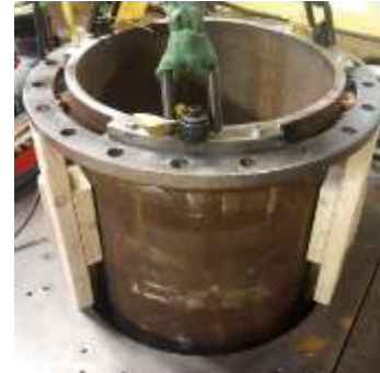
Temporary fixing of extension pipe with temporary support material (No.0)
