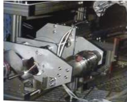
Connection of pipes
