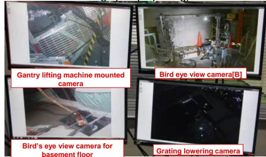
During work on the basement floor (after passing through pump opening)
