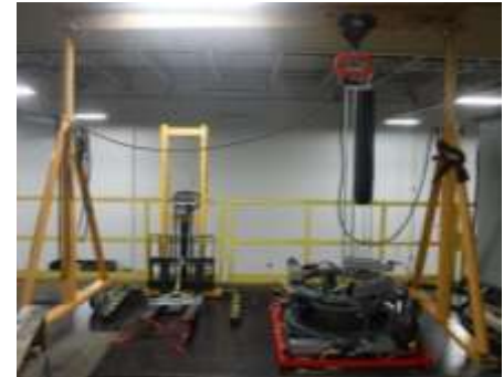
Installation of positioning tool (No.1)
