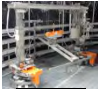
Transporting and installing the jigs
