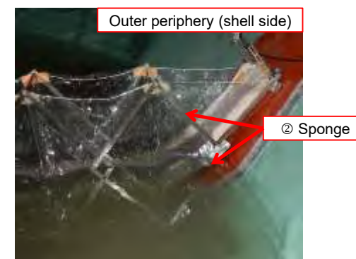
State of the weir on the outer periphery
