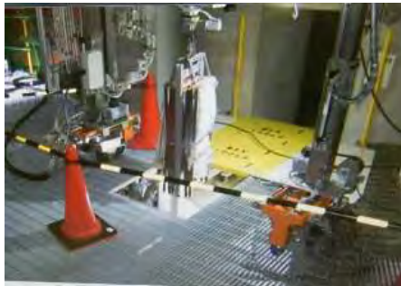
Carrying in formwork
