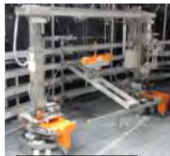
Transporting and installing the jigs
