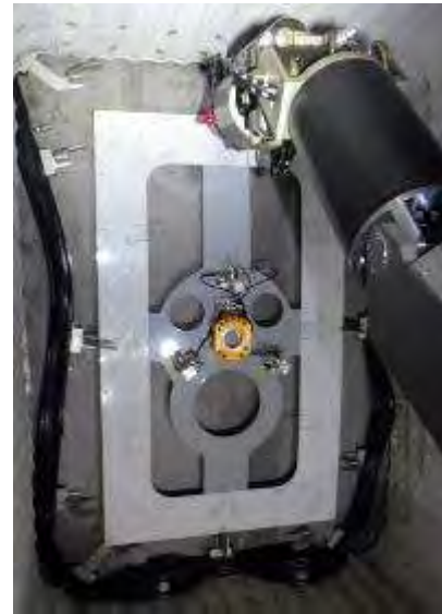
Insertion of inflate seal between gap
