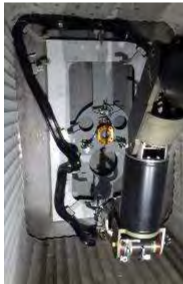
Temporary storage of inflate seal on PCV
