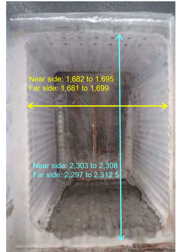
Opening part of BSW mock-up
