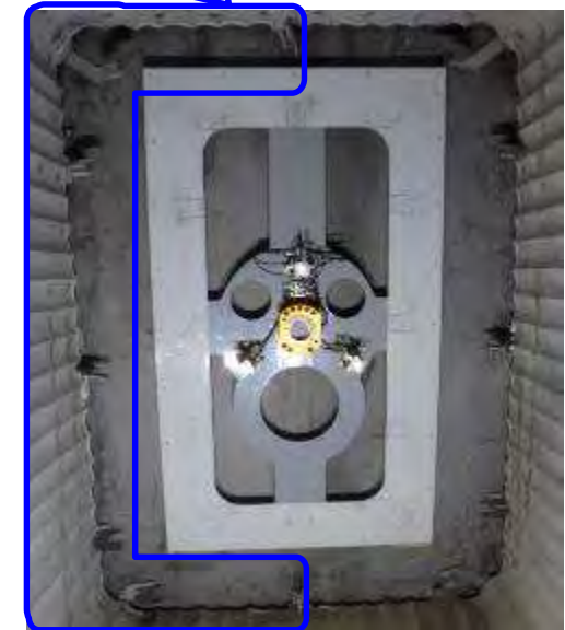
Completion of inflate seal installation
