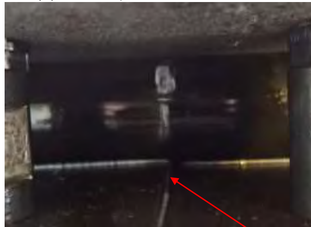
(e) Seal on joint of BSW mold
