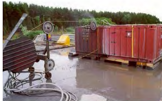
Cutting a solidified container
