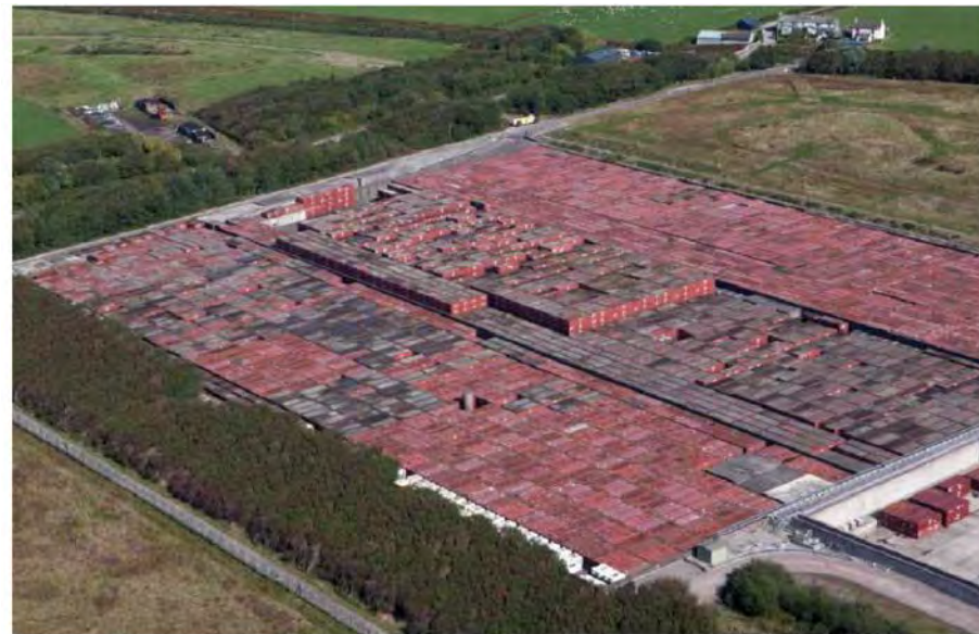
Containers of waste bodies placed at the LLWR disposal facility
