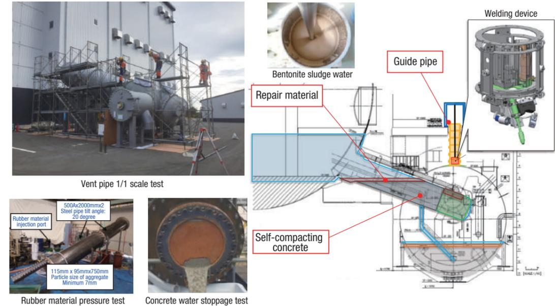
Figure: Overview of repairing lower part of PCV (filling in vent pipes and S/C guide pipe implementation)
