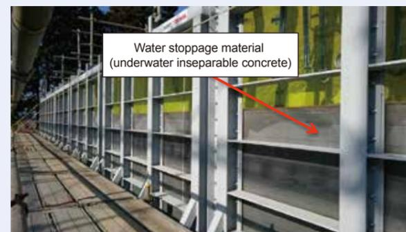
Fig. 3: Status of down-comer long-distance fluidity test
