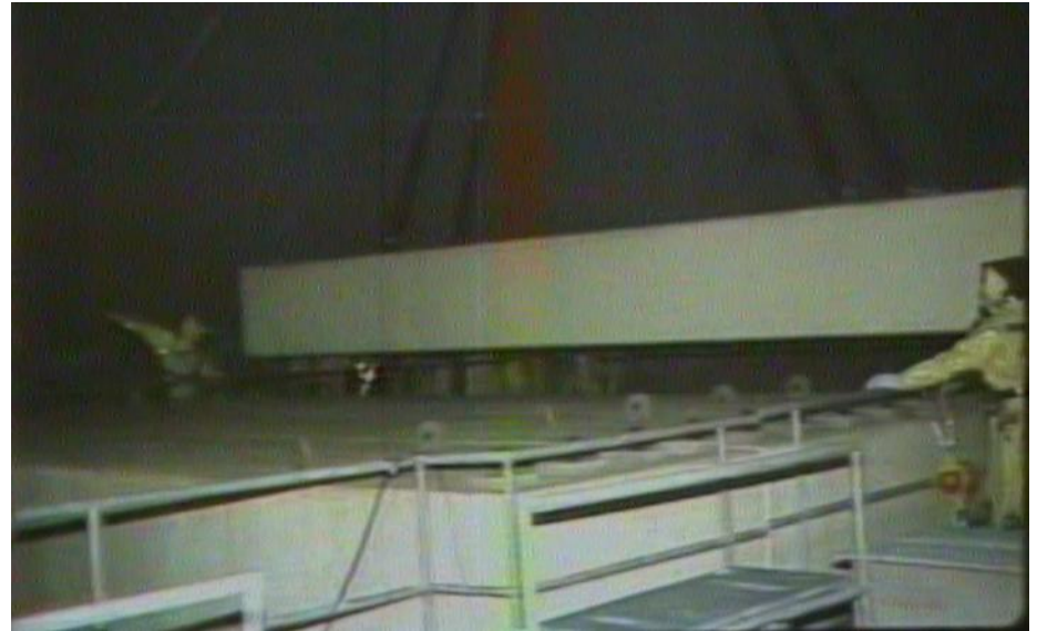
Lifting 40 Ton Missile Shield Blocks
