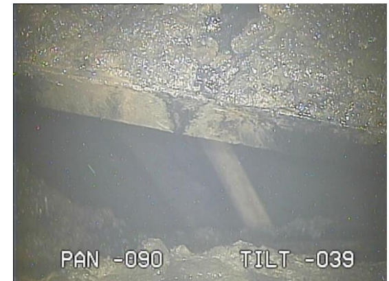
Gap between platform and CDR rail
